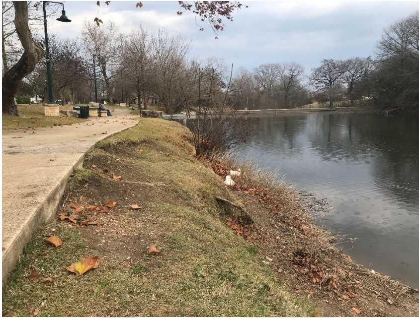
Soil erosion on creek side of sidewalk
