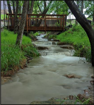
Example of natural channel design at Tanglewood Branch
