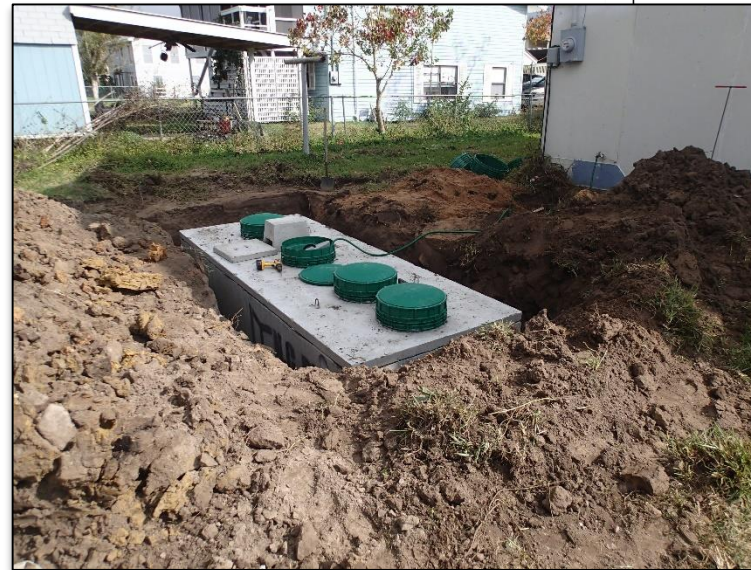
Example OSSF replacement; Photo credit Ryan Gerlich
