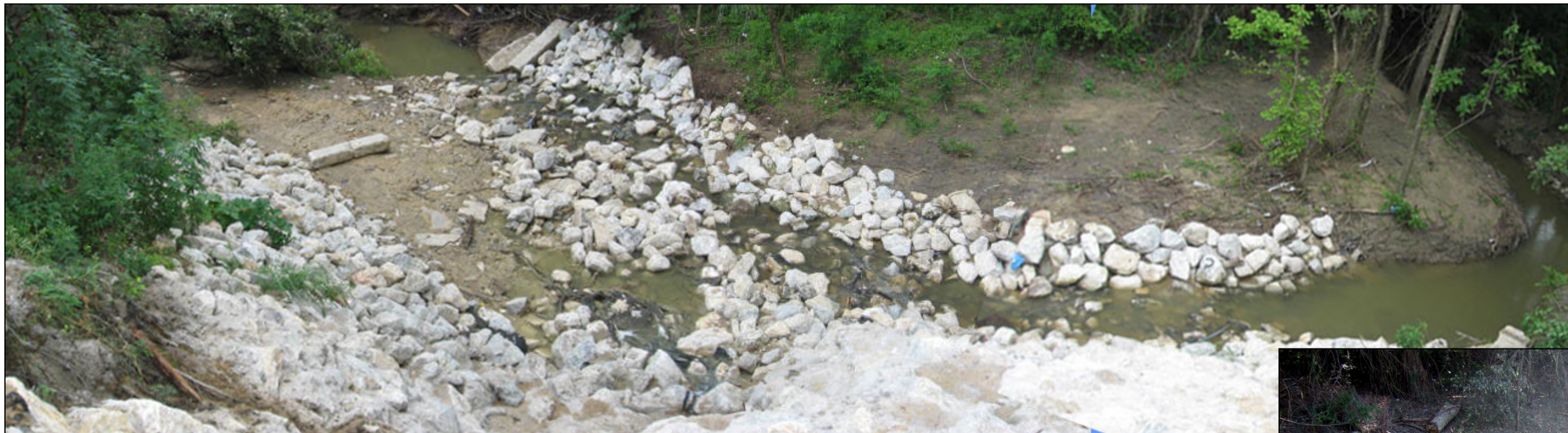
At 96" RCP Outfall near Christopher Drive
