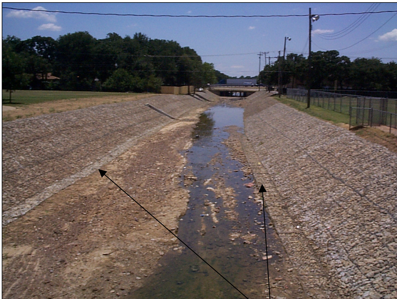
Notice 3'x3' toe wall (only top is exposed)
