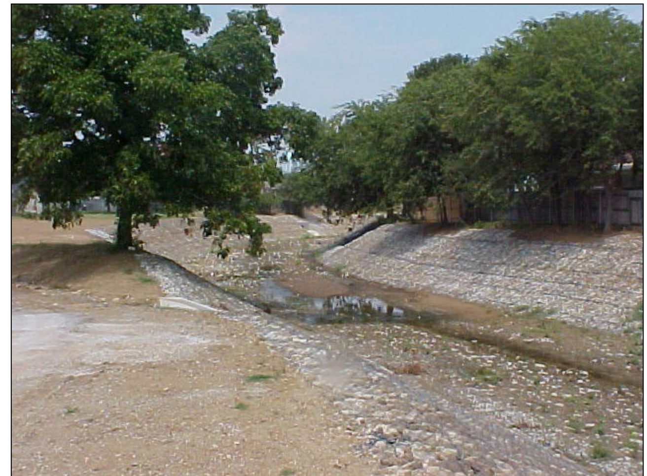
Gabion mattress side slopes
