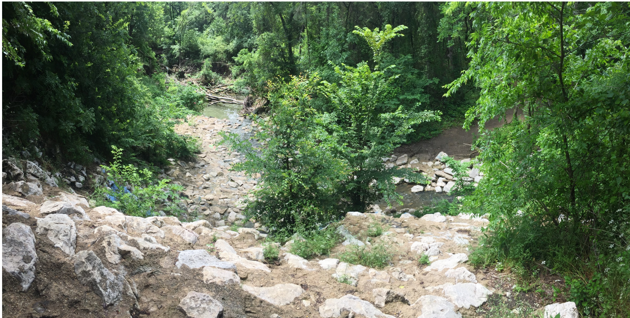
At 96" RCP Outfall near Christopher Drive
