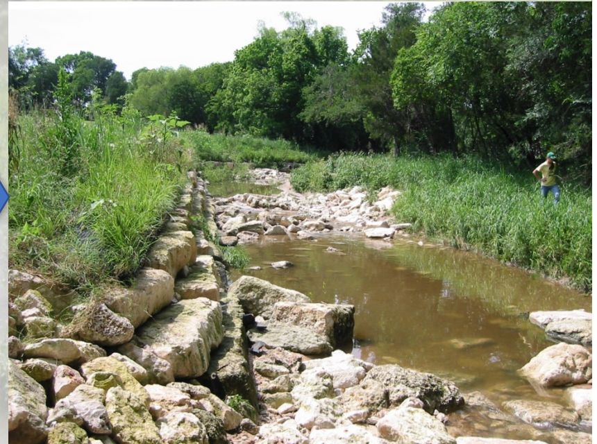
Restored - Good Condition
