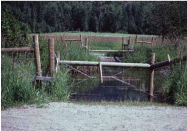
Figure 29. Narrow water access (water gap or gap) discourages loafing. (Photo by NRCS.)
