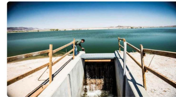
PROPOSED RUBICON POUROVER STRUCTURE WITH STOPLOG SLOTS
