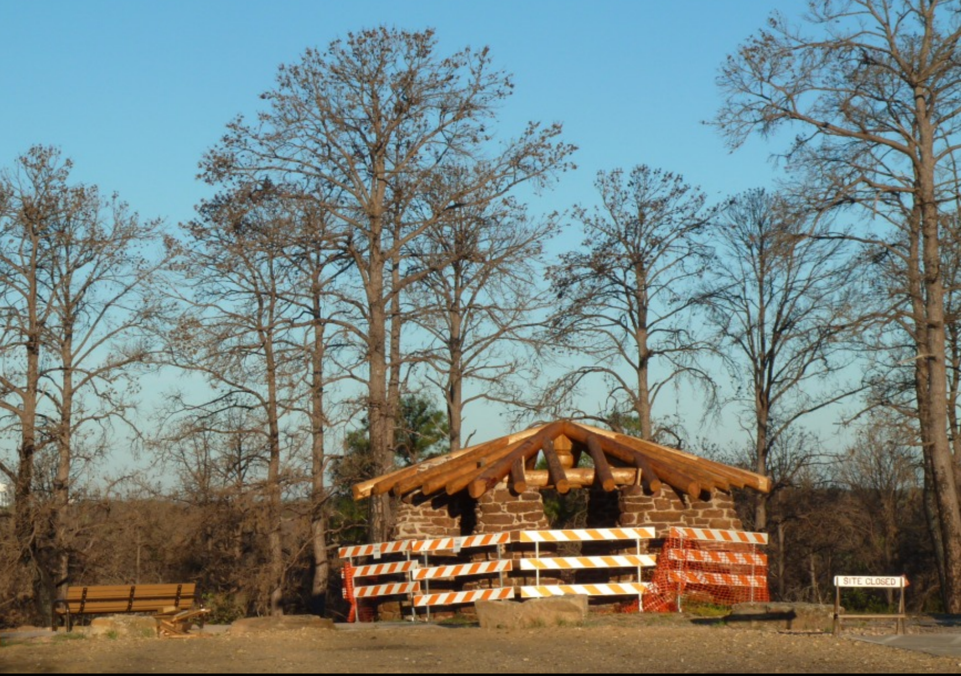
Scenic overlook shelter on Hwy 1A gets a new roof.
