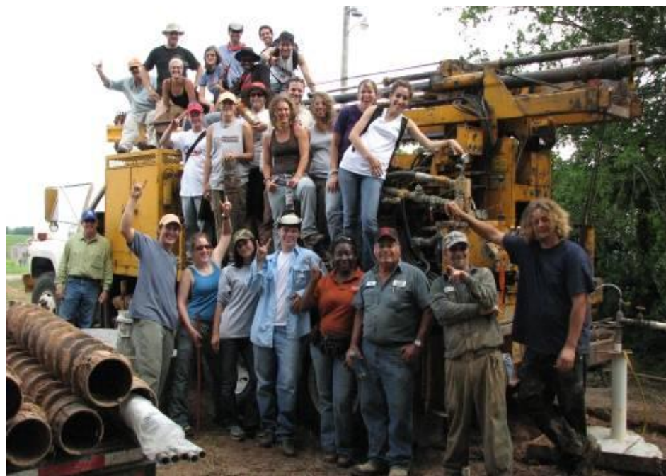
Group from UT Austin installing wells at Hornsby Bend.
